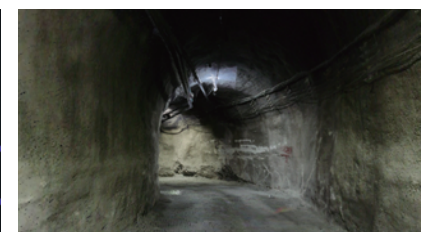
Mine Roadway colored Point Clouds
